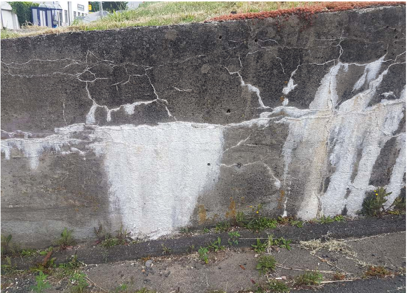
This retaining wall is permanently exposed to soil moisture. Leaking water has led to white efflorescence here.
