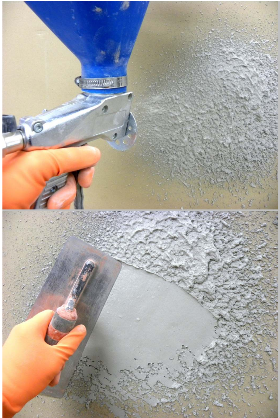
The funnel spray gun is very useful for applying the mortar easily and quickly to larger areas. The additives contained give the mass exactly the required consistency and stability. Smoothing is done with the smoothing trowel.
