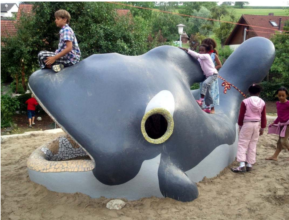
The whale house is a play and climbing object made of concrete. It was made of GRUMO basic mortar using the spraying technique and is lined with mosaic on the inside..
