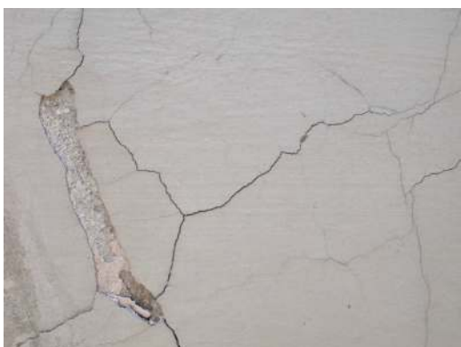
Shrinkage cracks are caused by stresses from the setting process. In the case shown here, the fault was that the hard surface layer was applied to a substrate that was too soft. Instead of absorbing the stresses from the setting surface layer, the soft substrate gave way. As a result, the surface layer cracked and came off.
