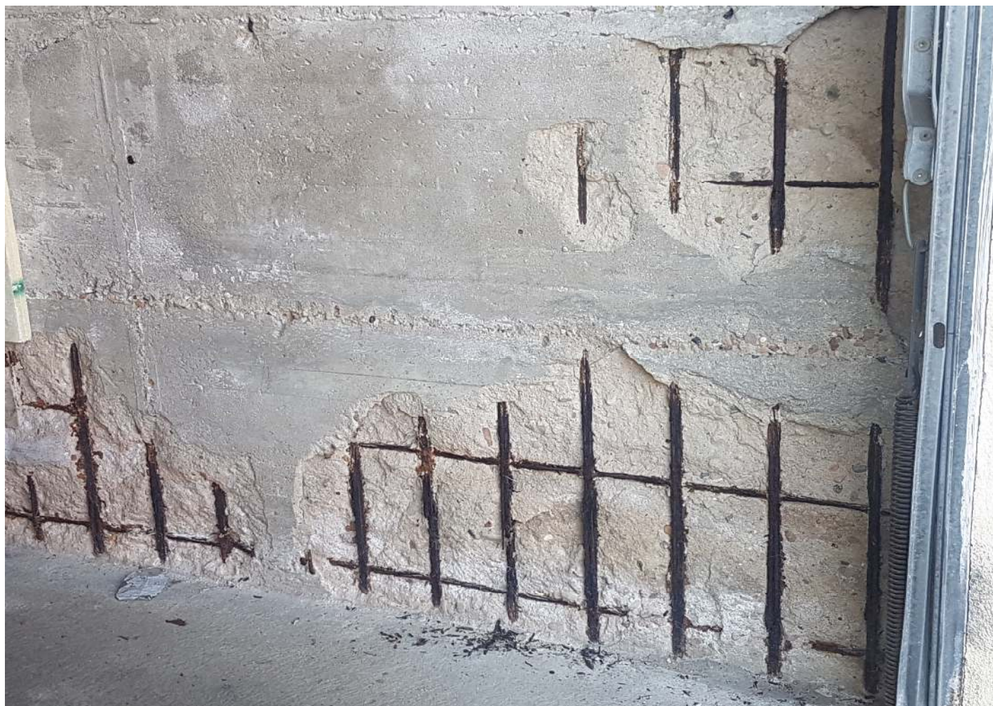
In this wall, the concrete cover is too small. This has allowed the steel reinforcement to rust and the top layer to blast off.
